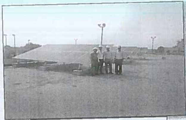
Solar PV Plant in DM Plant.
